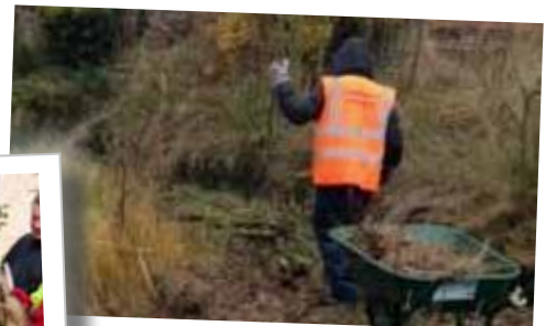
Ground clearing at Chicksands Army Base
